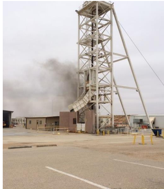
Figure 10: Smoke Visible Exiting through the Salt Shaft
