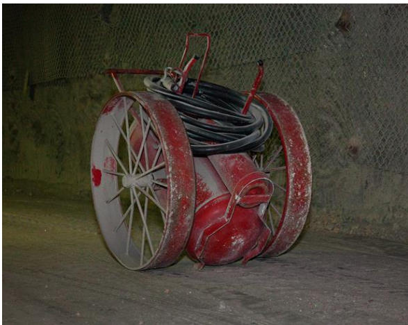
Figure 11: 300-Pound Extinguisher in the Underground
