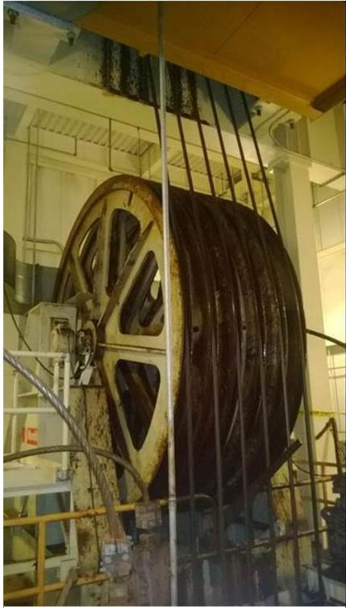
Figure 10: Waste Hoist Cable
