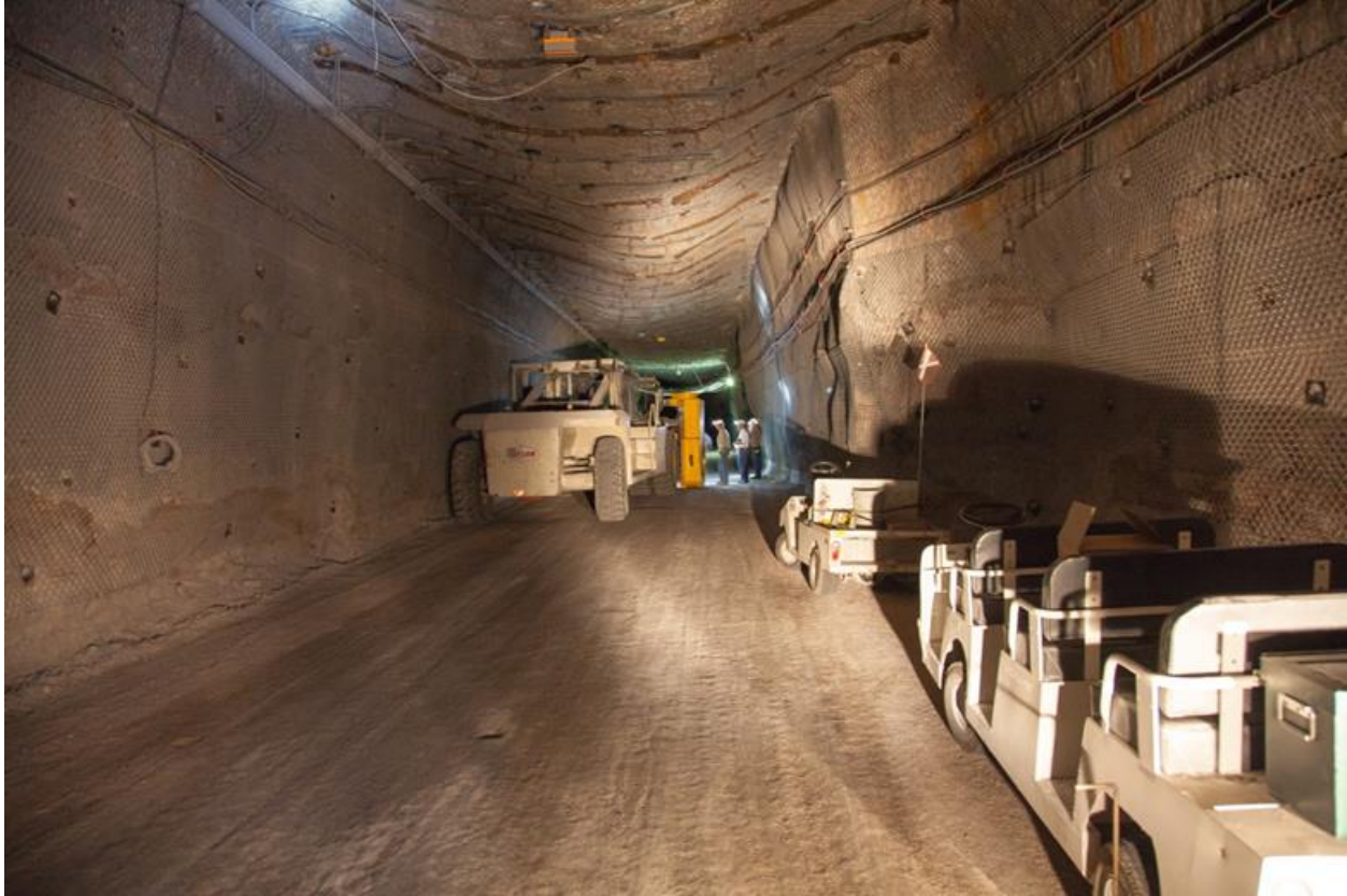
Figure 23: Ground and Rib Control in the Underground
