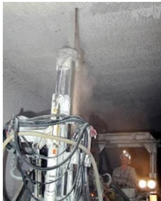
Figure 24: Roof Bolter Drilling to Install Roof Bolts
