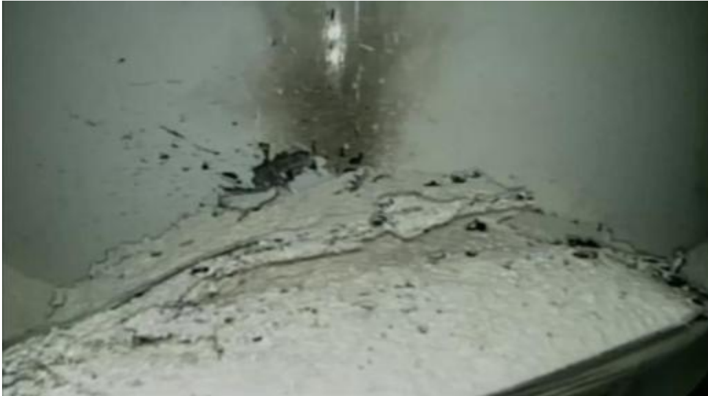
Figure 6-13: Face View (west) Base of Middle Tier Drum at R18:C6
