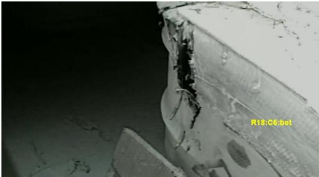
Figure 6-14: Face View (west) Stretch Wrap at Bottom Tier
