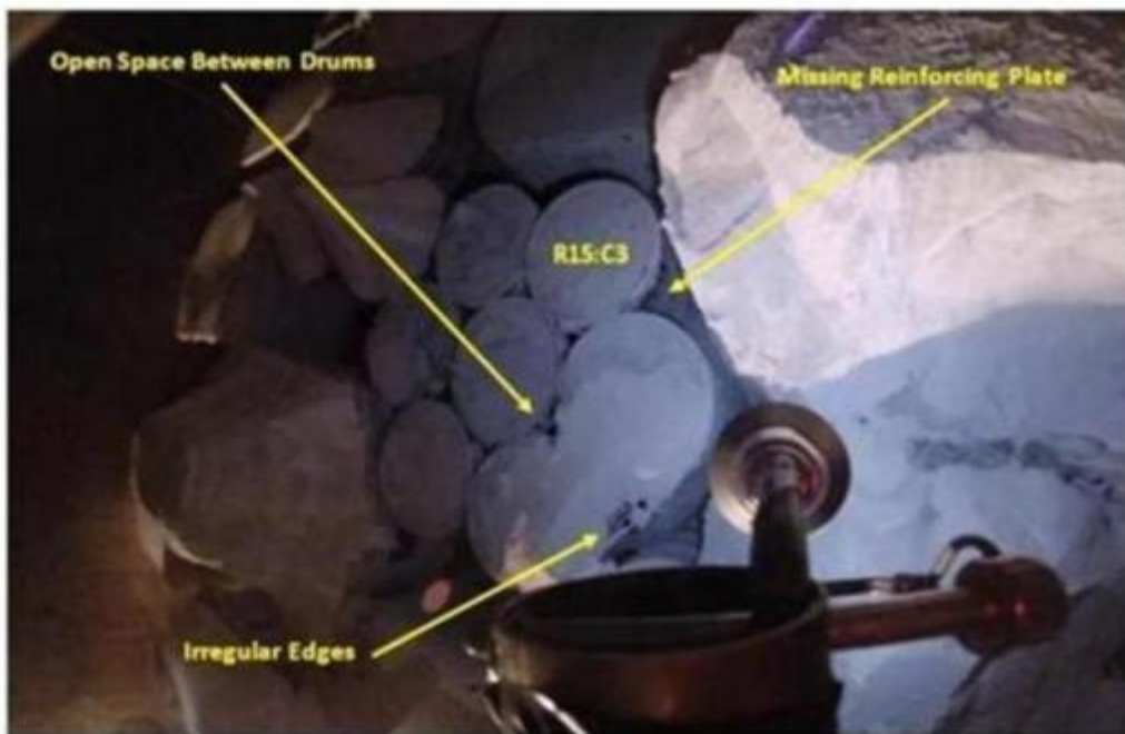
Figure 6-33: Missing Reinforcement Plate at R15:C3
