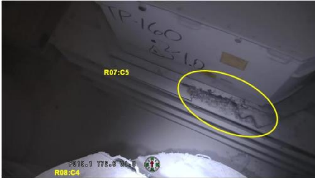
Figure 6-10: Fiberboard Slip Sheet Damage at R7:C5
