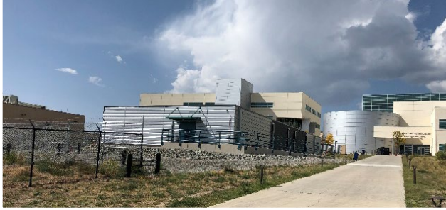
Secured office facility: complete
