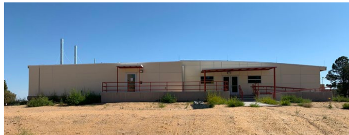
Bio lab & office facility: complete
