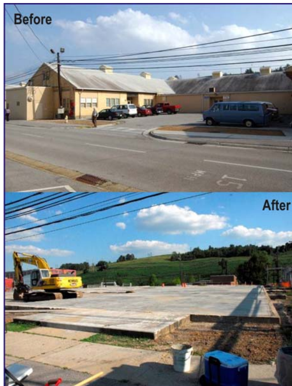
Figure 11-3. Demolition of Building 9734 at Y-12 was completed in September 2008.
