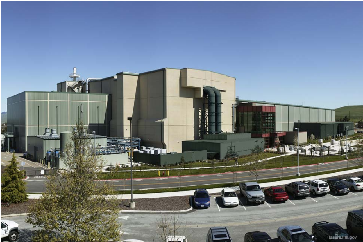
Figure 5-2. The National Ignition Facility was completed in the second quarter of FY 2009.
