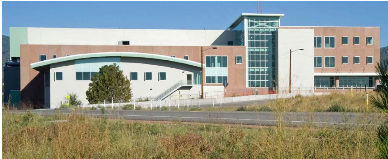
Figure 2–3 Radiological Laboratory/Utility/Office Building in Technical Area 55
