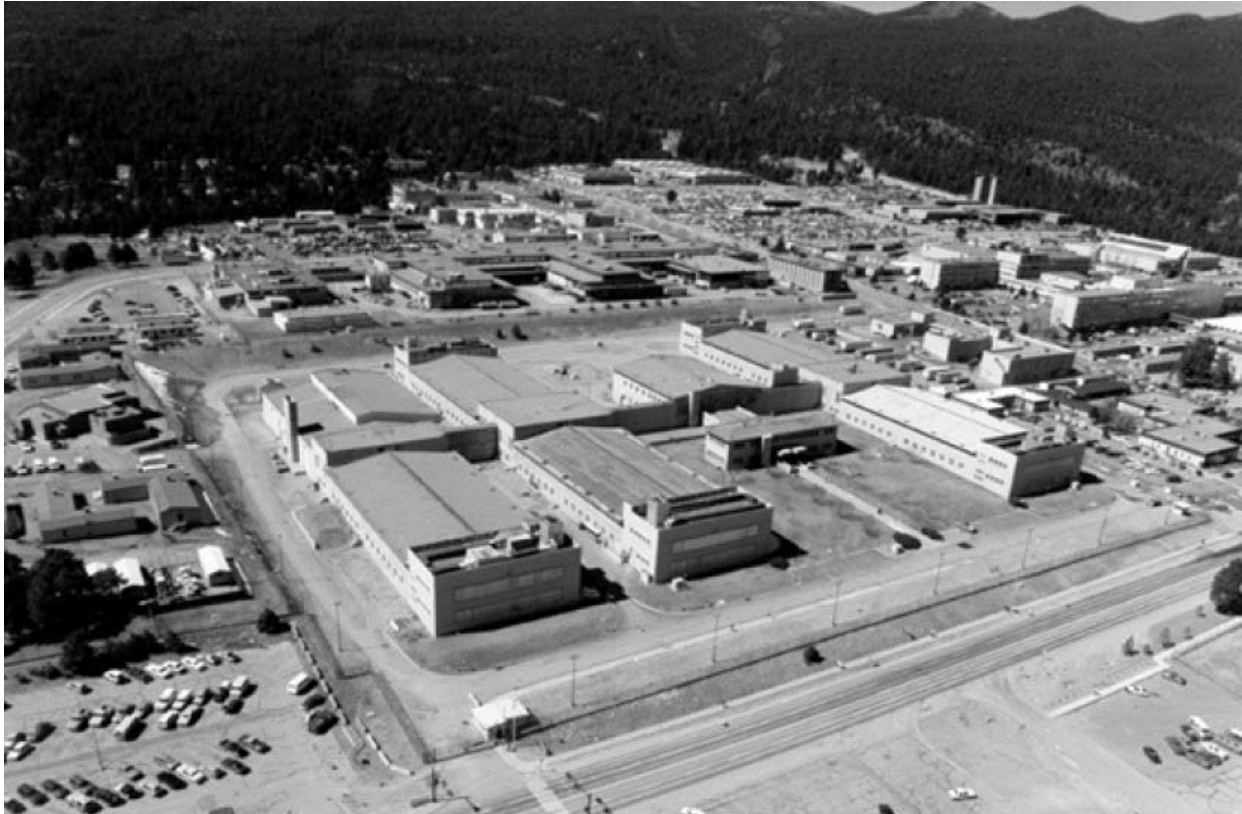
Figure 2–1 Existing Chemistry and Metallurgy Research Building
