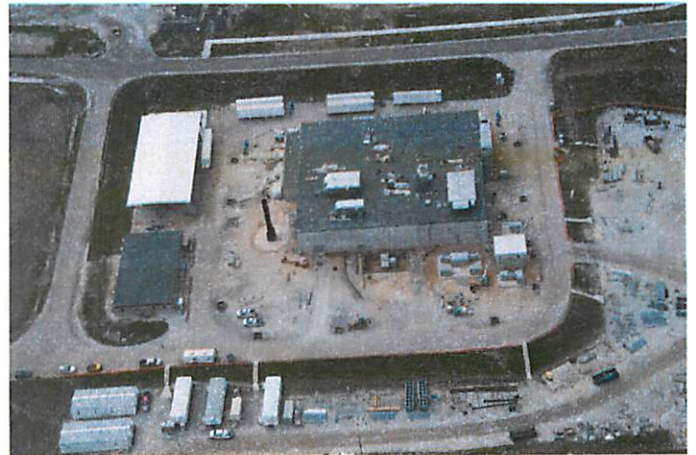
Figure 5-7: Waste Solidification Building (March 2012)
