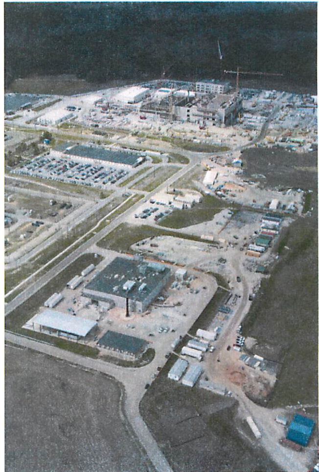
SRS Nuclear Nonproliferation Facilities Under Construction (March 2012)
