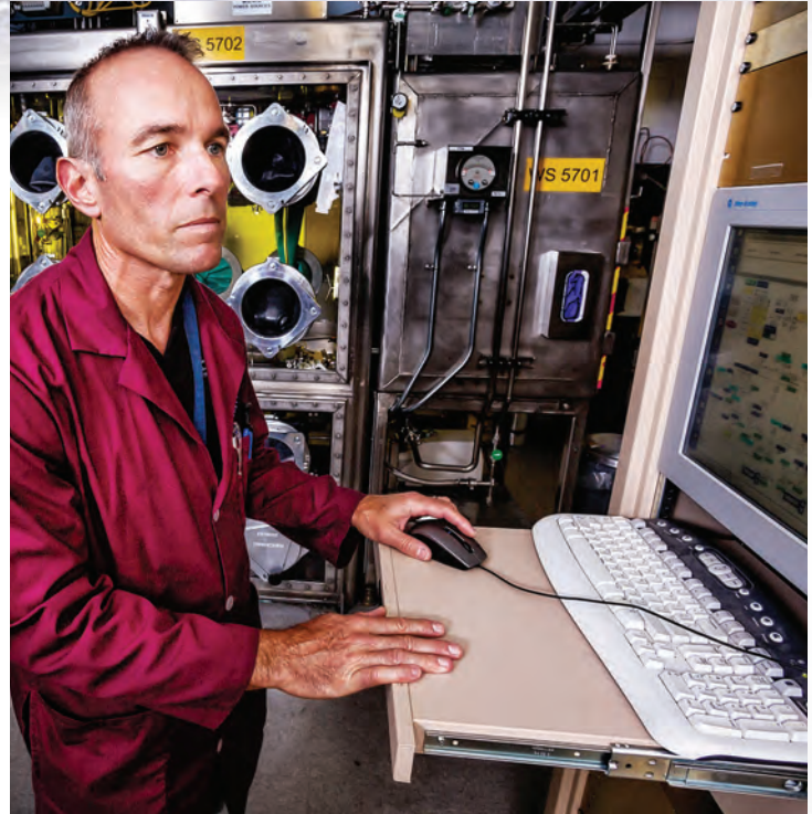
Tritium processing station and recovery system.
