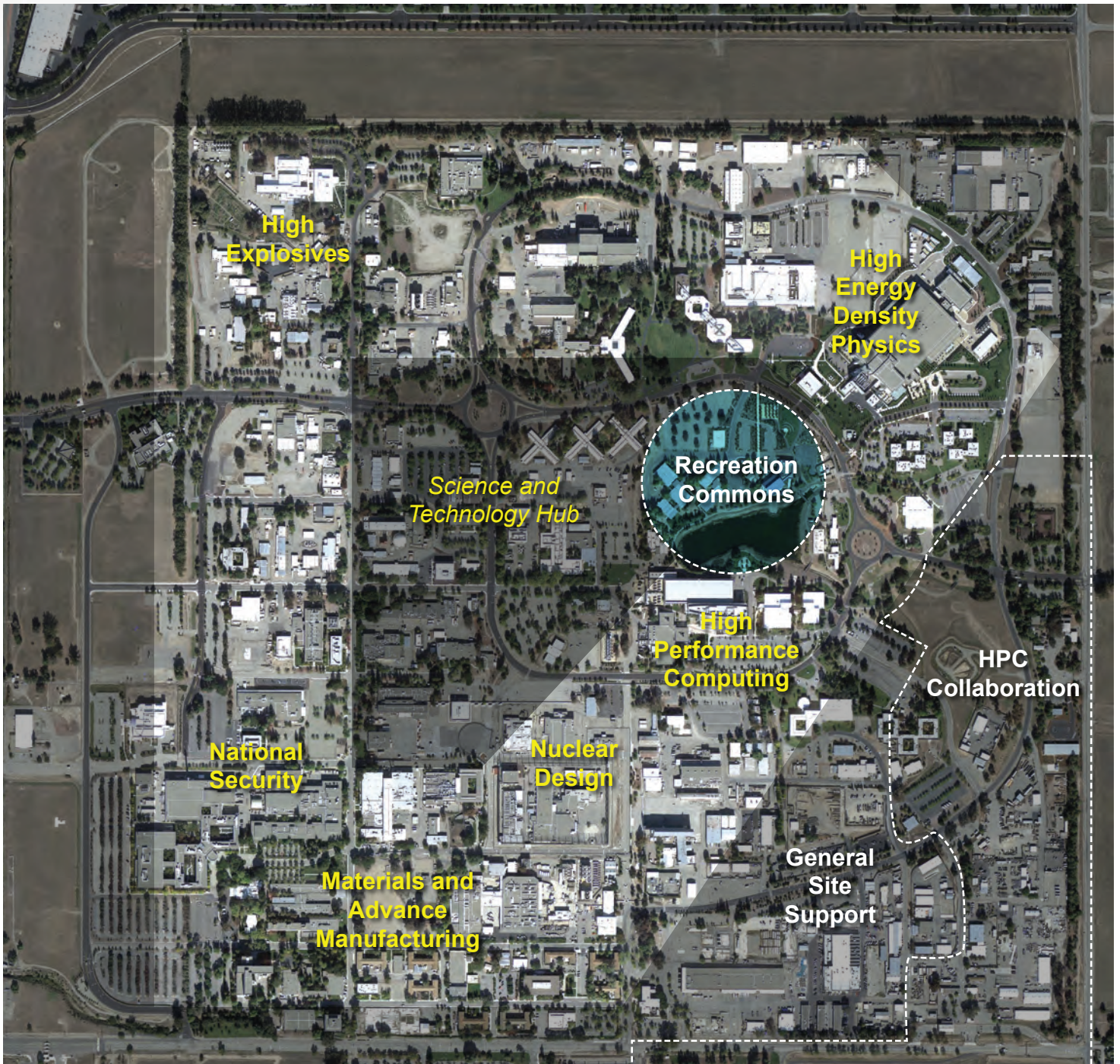
Strategic site planning for redevelopment envisions Program-corridors, linking existing signature core capabilities and future Program project sites; and in the center would be a multi-disciplined science and technology hub of sharable resources to reduce duplicity. The southeast quadrant of the site is reserved for general site support and connects with open collaboration initiatives.
