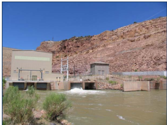
Figure 2: Abiquiu Hydro Electric Power Plant
