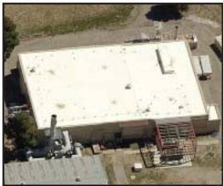
Beryllium Technology Facility (BTF)
