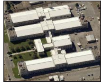
Chemistry and Metallurgy Research (CMR) Facility
