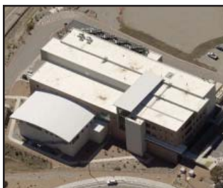
Radiological Laboratory Utility Office Building (RLUOB)
