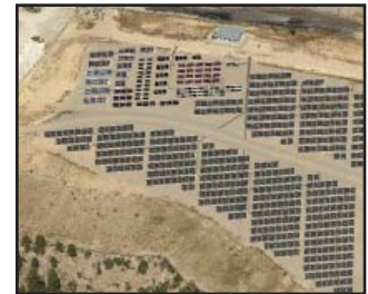
Photovoltaics at TA-61 (landfill)
