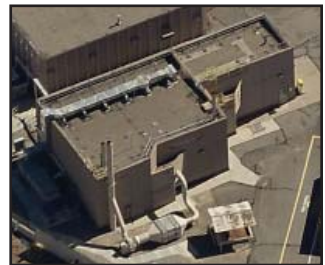
Waste Characterization, Reduction, and Repackaging (WCRR) Facility
