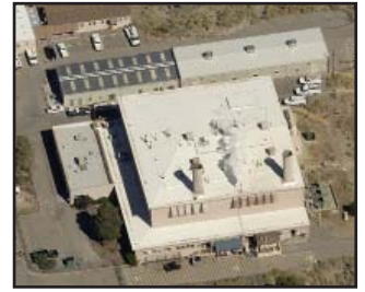
Steam Plant at TA-3
