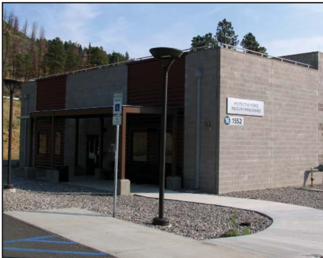
Protective Force Indoor Firing Range at TA-16
