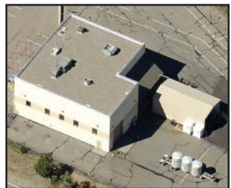
Radioactive Assay Nondestructive Testing (RANT) Facility
