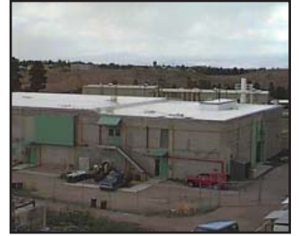
Beryllium Technology Facility (BTF)
