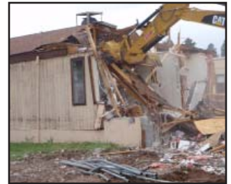
D&D of Temporary Structures
