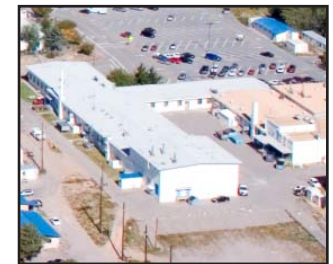
Aging/Obsolete Laboratory at TA-35-0002
