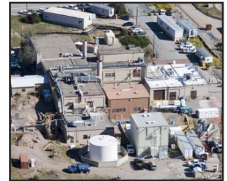
Radioactive Liquid Waste Treatment Facility (RLWTF) Upgrades
