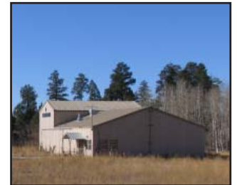
Aging/Obsolete Facility at Fenton Hill
