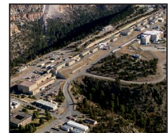
Proposed Stand-off Active Interrogation Field Site and Proton Interrogation Facility at LANSCCE
