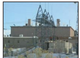
Replacement of the TA-3 Steam Plant
