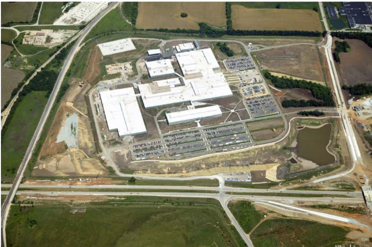
Figure 4: Botts Road Site Construction Progress as of June 05, 2012
