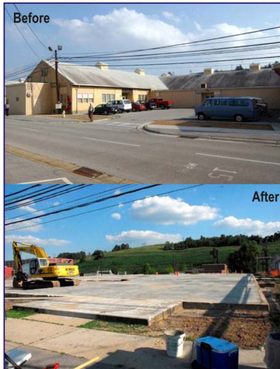
Figure A-11-3. Demolition of Building 9734 at Y-12 was completed in September 2008.
