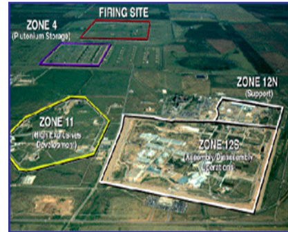
Pantex Plant Amarillo, Texas Weapons assembly/disassembly
