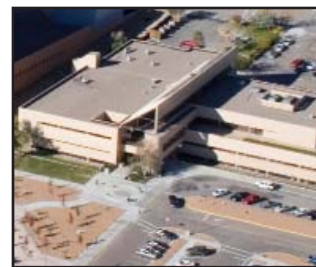
Otowi Building Life Extension Project
