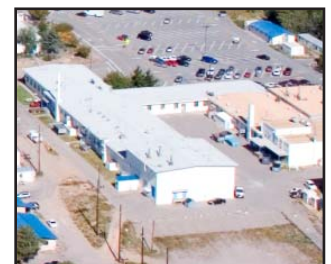
Aging/Obsolete Laboratory at TA-35-0002
