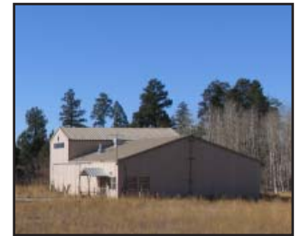
Aging/Obsolete Facility at Fenton Hill
