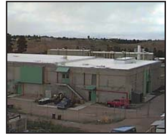
Beryllium Technology Facility (BTF)
