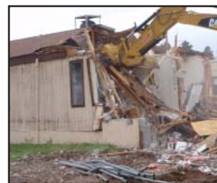
D&D of Temporary Structures
