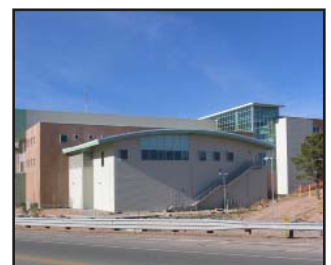
Radiological Laboratory Utility Office Building (RLUOB)
