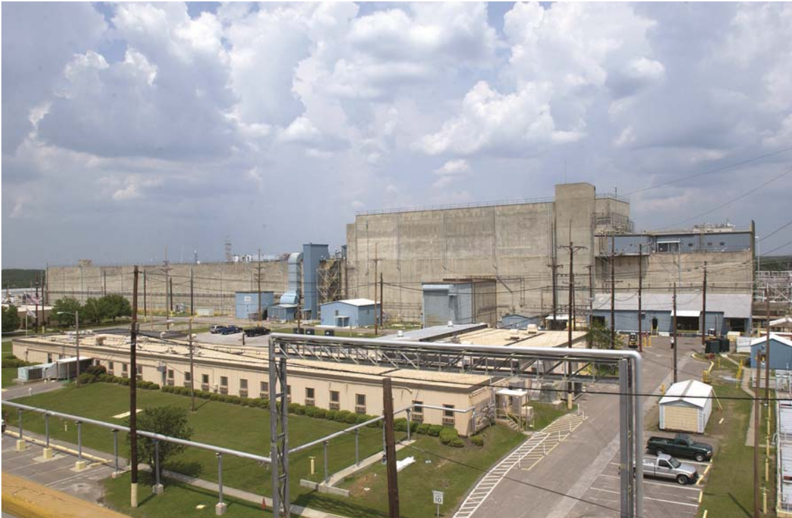
Figure E4: H-Canyon and HB-Line Processing Facility
