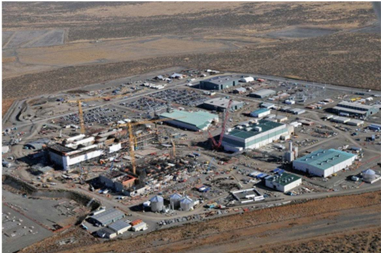
Figure E1: Hanford Site - Waste Treatment and Immobilization Plant under Construction
