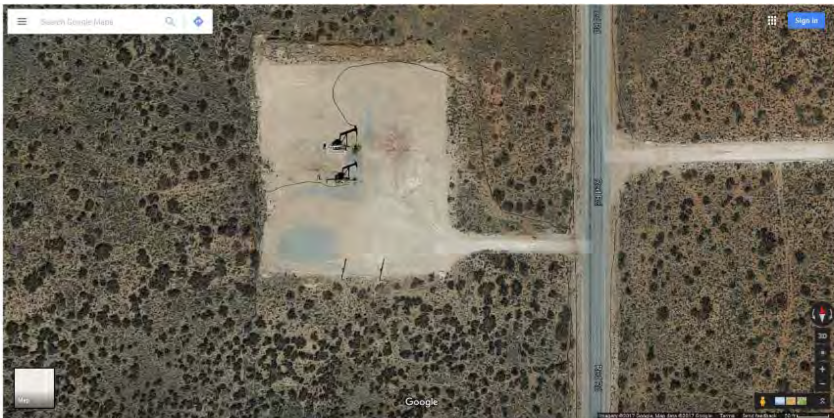
Figure D-29. Oil well near WIPP
