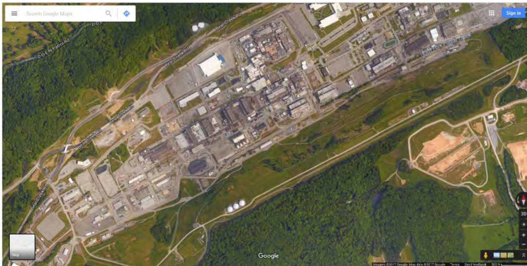
Figure D-24. Close-up of SW end of Y-12 showing PIDAS
