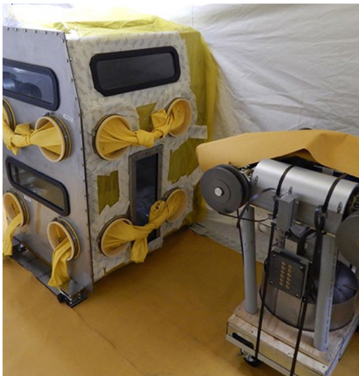
In 2020, upgrading the aging trolley system at the Plutonium Facility was a priority for the Weapons Infrastructure Program Office.
