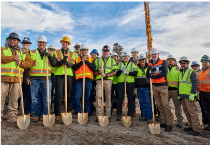
In February 2020, Laboratory leaders and contractors held a groundbreaking ceremony for a new cell tower at TA-15.
