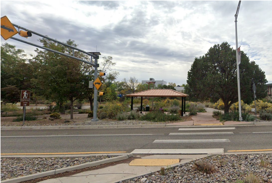
Figure 43 SR4 & Sherwood Bus Shelter
