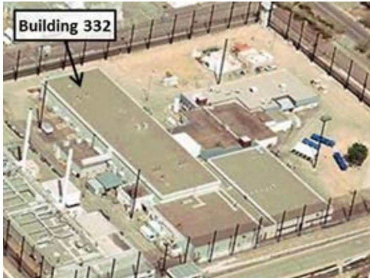
Building 332 Source: Lawrence Livermore National Laboratory
