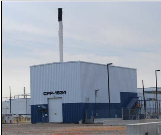
Figure 7. Building CPP-1634 At Idaho National Laboratory
