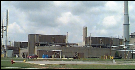
Figure 10. F/H Laboratory At Savannah River Site
