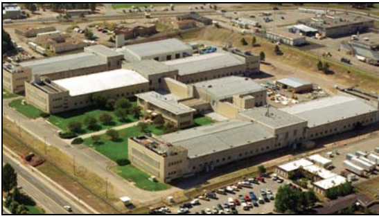
Figure 3. Chemistry and Metallurgy Research Building
