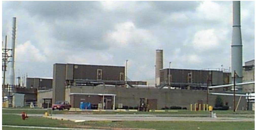
F/H Laboratory Source: Savannah River Site
