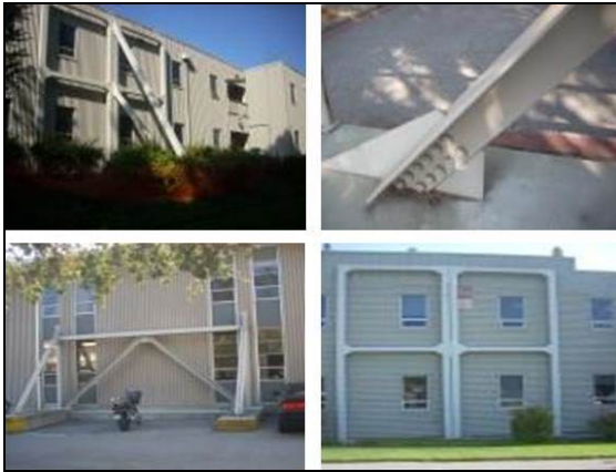
Figure 13. Seismic Bracing of Office Buildings
