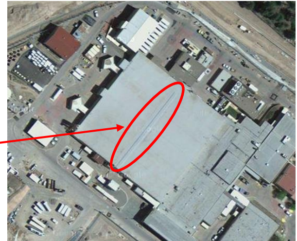
Photo: Google Maps. Photo shows PF-4 roof with drag strut circled.
