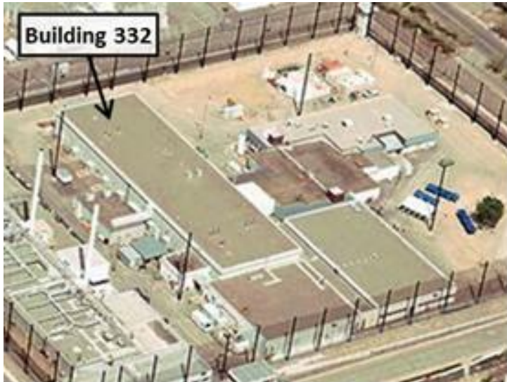
Building 332 Source: Lawrence Livermore National Laboratory
