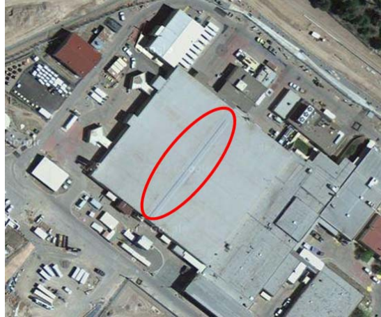
Figure 5. PF-4 Roof Showing Drag Strut Drag strut is circled
