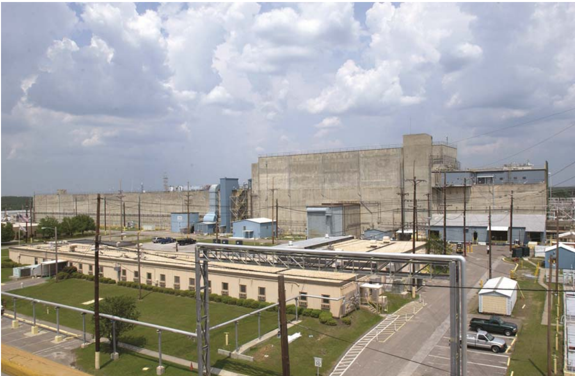
Figure E4: H-Canyon and HB-Line Processing Facility
