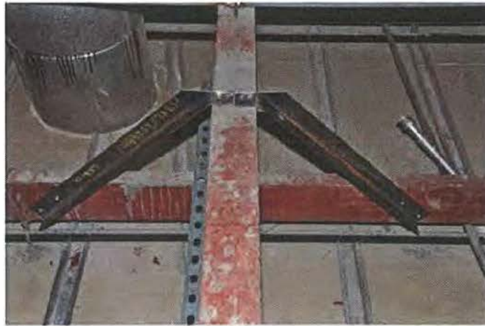
Figure 3. Ceiling Beam Brace from Top of I-beam to C-channel
