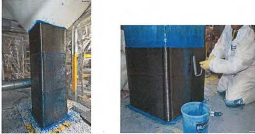
Figure 5. Basement Column reinforcement
