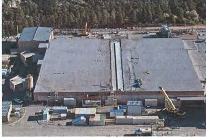
Figure 1. New Drag Strut Across PF-4 Roof
