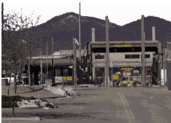
The entrance to the TA-55 Plutonium Facility.
