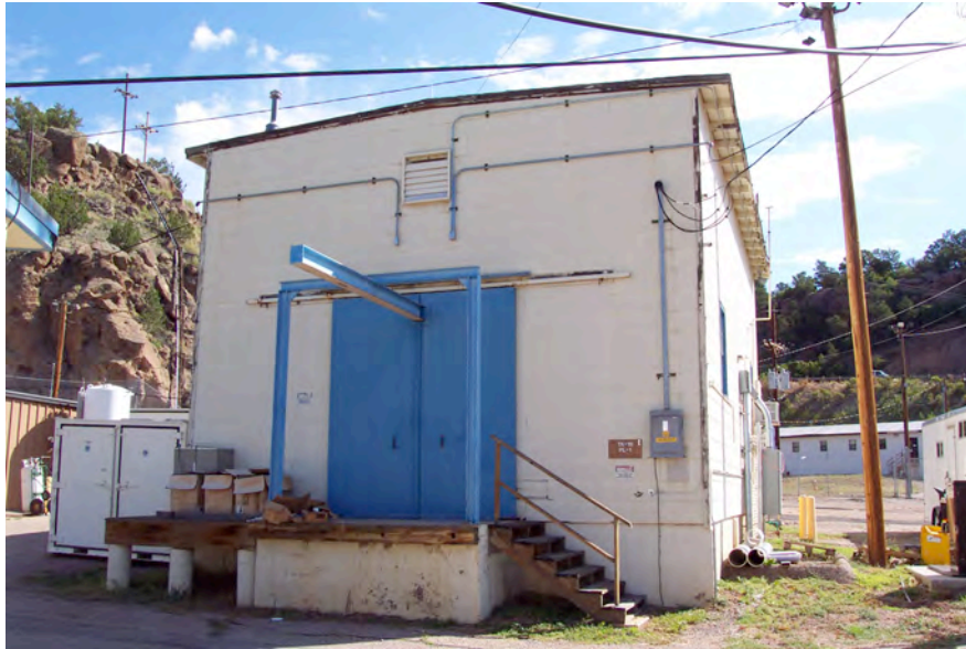
Figure 15.9. Building 18-1, site of a fatal criticality accident.
