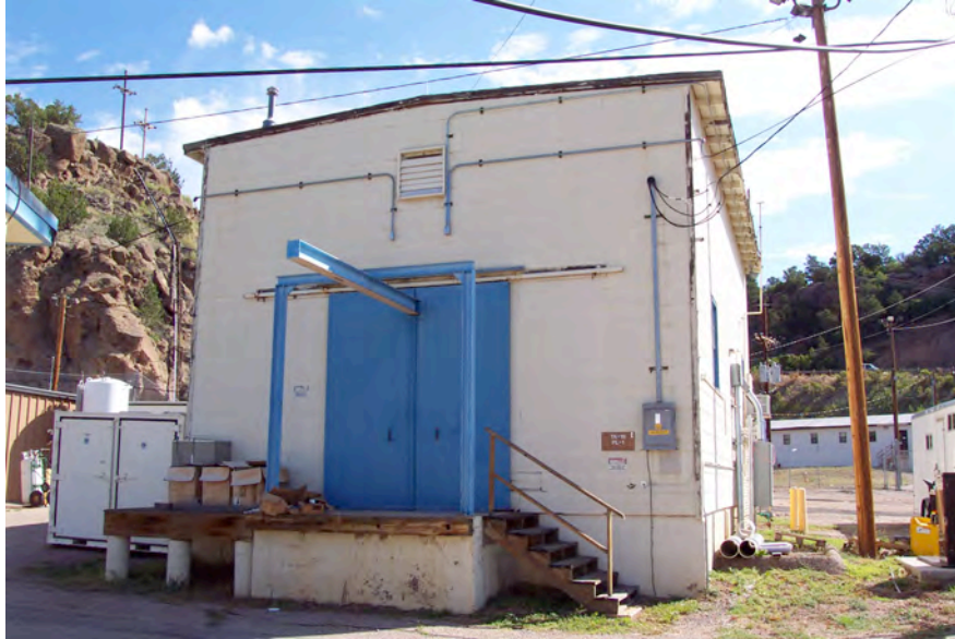
Figure 15.9. Building 18-1, site of a fatal criticality accident.
