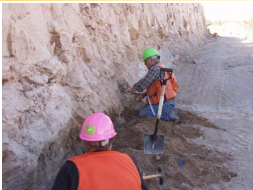
▲ Clearly exposing geologic features on excavation wall in preparation for further analyses
