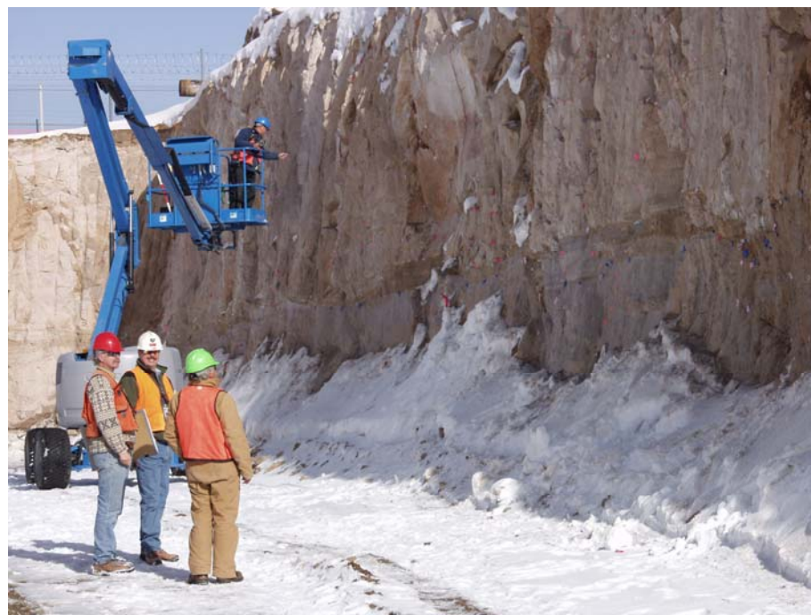
Logging and surveying temporary excavation walls, January 2007
