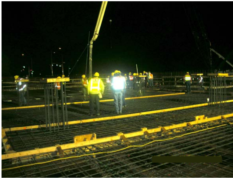
#2559 - RLUOB Status Looking Southwest
